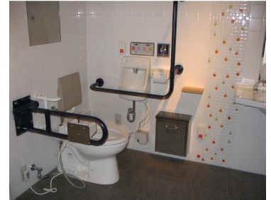
An accessible TOTO toilet in Japan.
